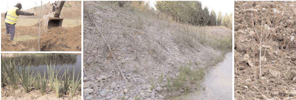
Figure 13. Different planting techniques used in the Mink Territory project. Bare-root planting, Salix cuttings on banks and coir logs with helophytic species on banks.
