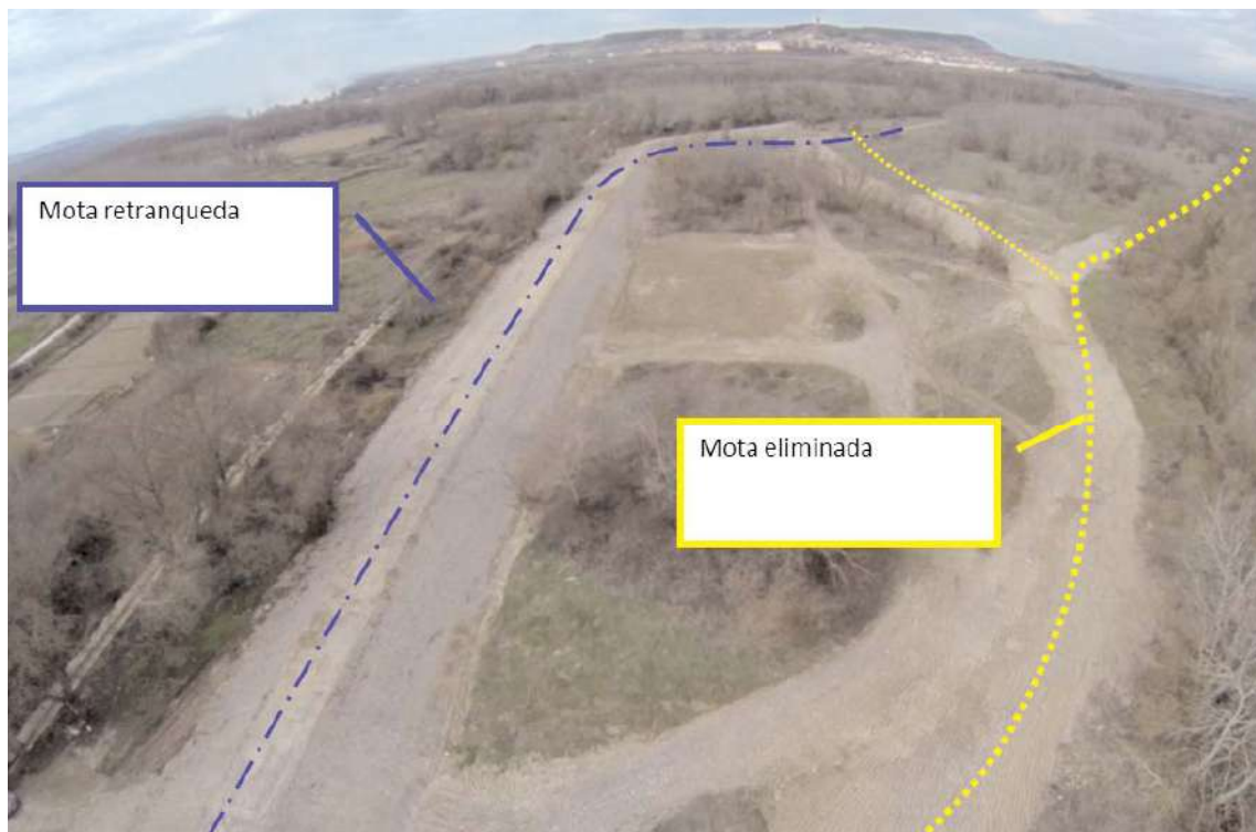
Figure 3. Earth embankment set back in Soto Sequero (Mérida), gaining 11.62 hectares for the Aragon River and, consequently, returning a certain degree of river activity to riparian woodland which was lacking in this regard.
